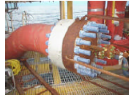
16" 1500 Taper-Lok Riser Flange & Test Blind
