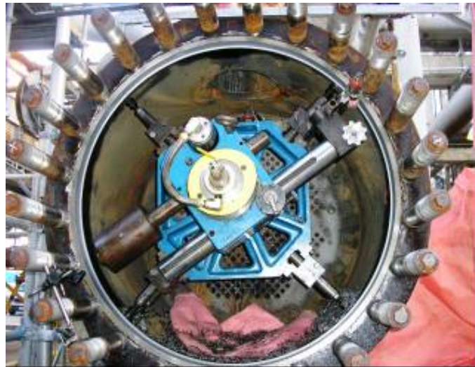
Figure 6 - Machining pressure seal female pocket with ID mounted tool
