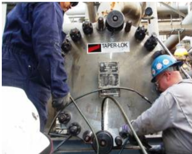
Figure 8 - Hydraulic tensioning and installation of mechanical tensioners
